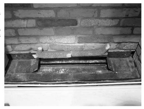
Place a further 2 off log shapes along the front edge of the burner cover as shown.
