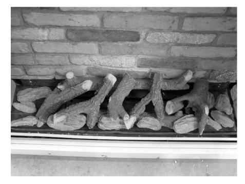
• Place the last Two large shapes LH and RH as shown.
